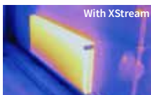
Radiator without air or dirt
